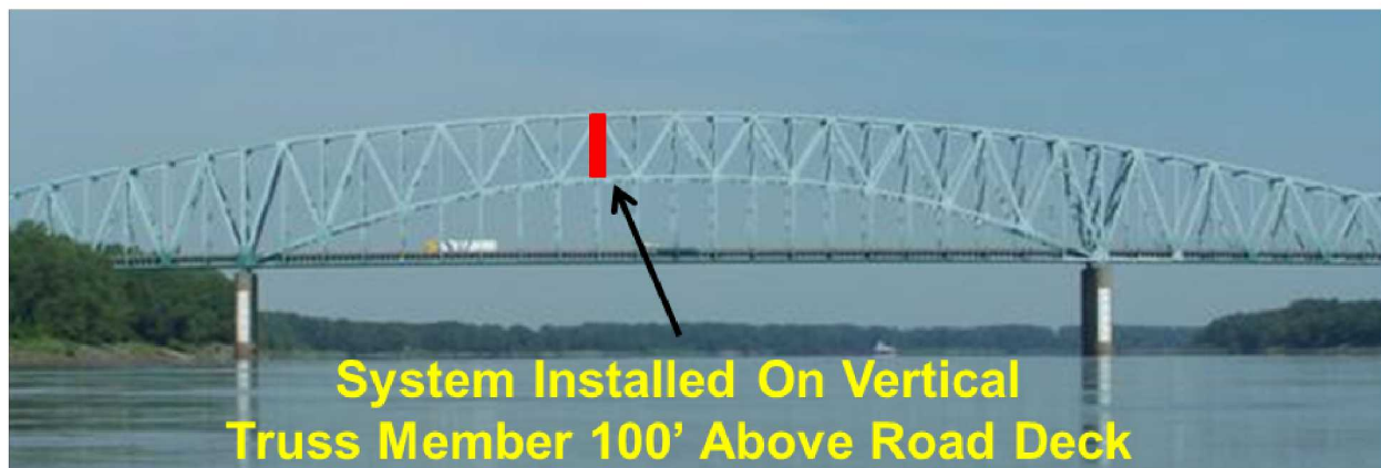
Figure 2-15: Placement of CVM Sensor Network for Monitoring Critical Bridge Welds
