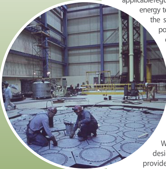
Refueling floor at Fort St. Vrain Generating Station, one of the first HTGR power reactors in the U.S.
