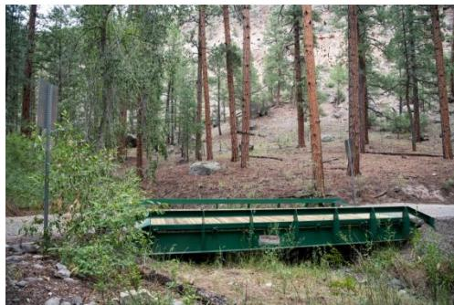
**Photo Caption:** This photo presents a side view of new, stronger bridges designed to handle 28-ton firefighting tankers with loads full of water.
