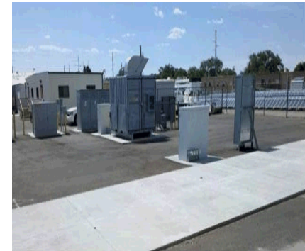
The new 1 MW Energy Storage Test Bed integrated with renewable energy generation at Sandia's Distributed Energy Technology Laboratory.
