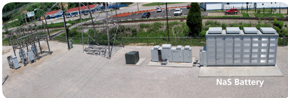
This Sandia-led DOE Office of Electricity demonstration project proved the effectiveness of sodium-sulfur batteries in peak shaving and capital deferment.
