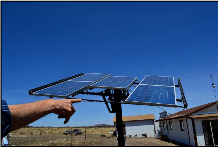
Ground mounted solar PV system on residential unit in Grand Falls, AZ
