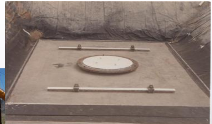
Concrete pad at bottom. Anchor points and extension cover shown
