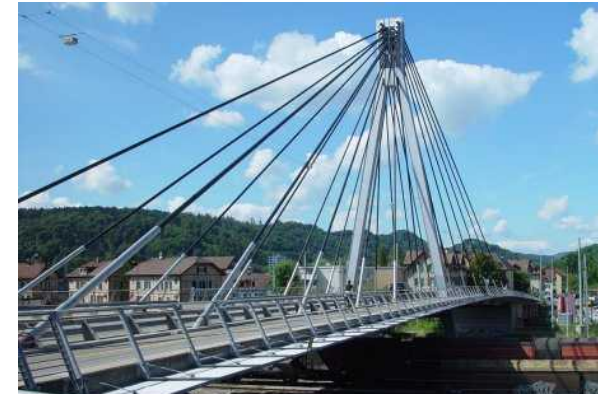
CFRP cable stay bridge
