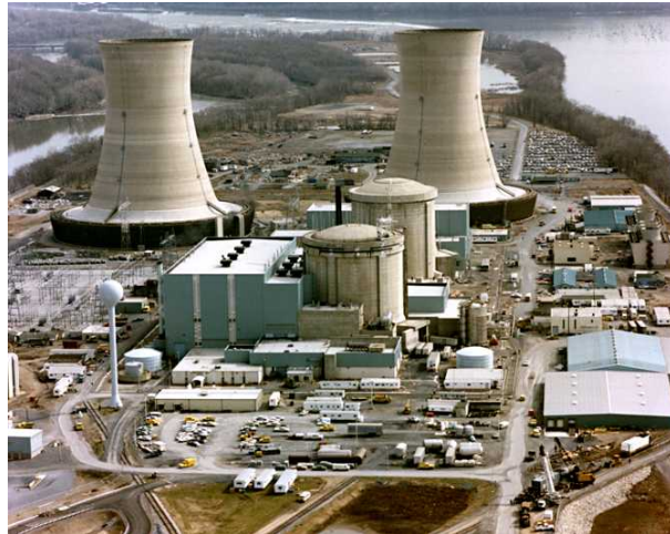
Nuclear Power Plant Cable Insulation
