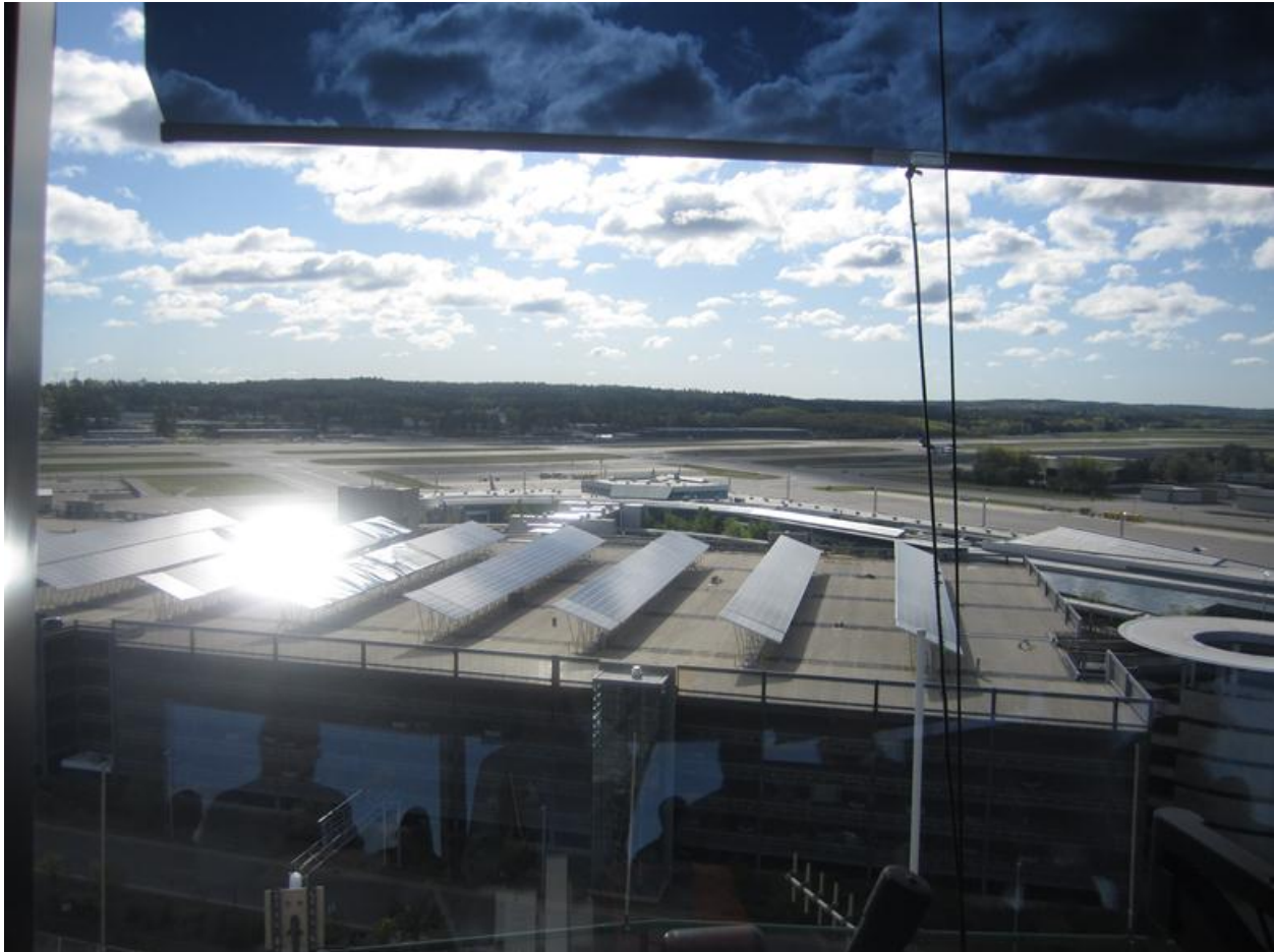
Figure 12. Glare viewed from Air Traffic Control Tower at Manchester/Boston Regional Airport (~8:17 AM EDT, 5/10/12). Note that tarp has been placed over some of the modules.
