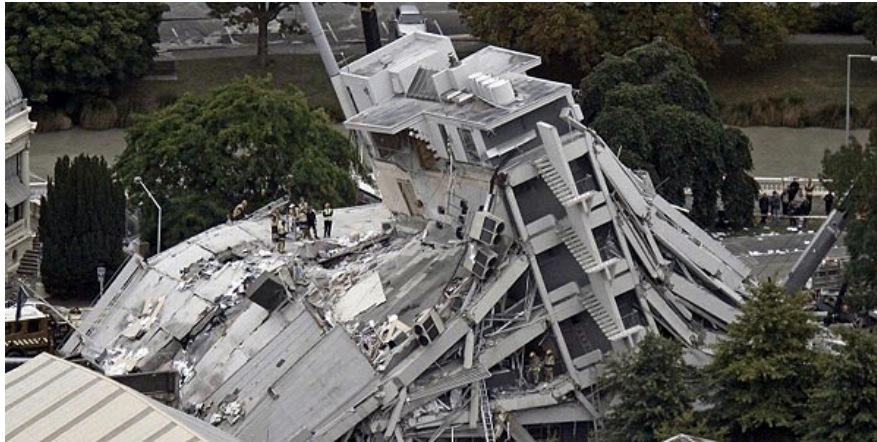
2010 New Zealand Earthquake (7.2 Magnitude)
