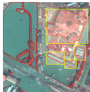
Figure 1. An example RS image showing building regions strongly flooded from west direction. Regions are delineated with red color and their corresponding MBRs are shown with yellow border. (Image source: WV2, Srinagar, India, Flood event 2014).
