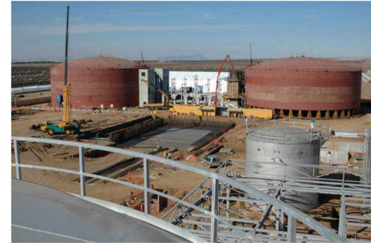
50MW AndaSol-1 Parabolic Trough Plant w/ 7-hr Storage Andalusia, Spain
