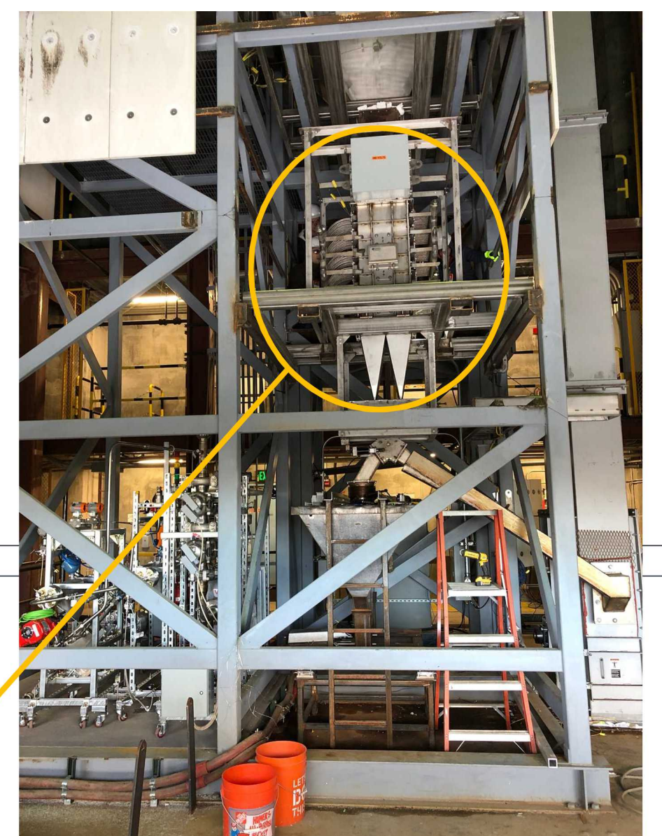
Solex/VPE/Sandia particle/sCO 2 shell-and-plate heat exchanger
