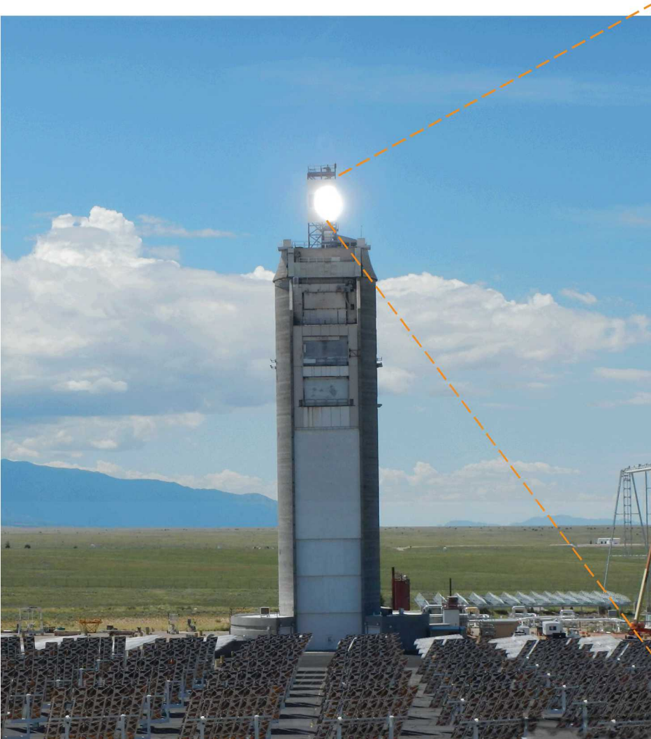
Particle receiver testing at the National Solar Thermal Test Facility at Sandia National Laboratories, Albuquerque, NM
