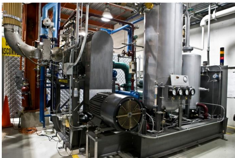
Figure 4: 12 g/s KMDB10000/Pompe ring pump combination
