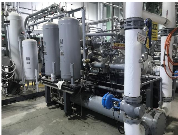
Figure 1: Typical Mycom compressor with Oil removal
