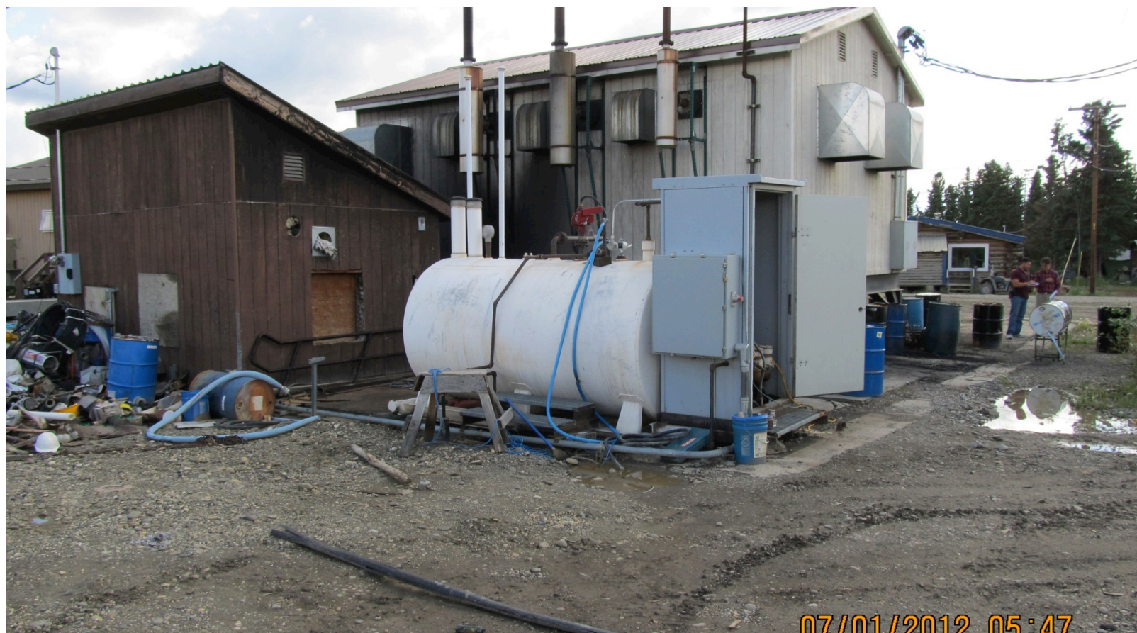
Venetie Generator building with 1500 gallon fuel tank in foreground
