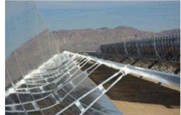
SkyTrough® with ReflecTech® Mirror Film (SEGS II)
