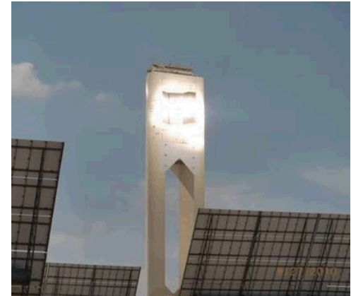
Cavity tubular receiver
