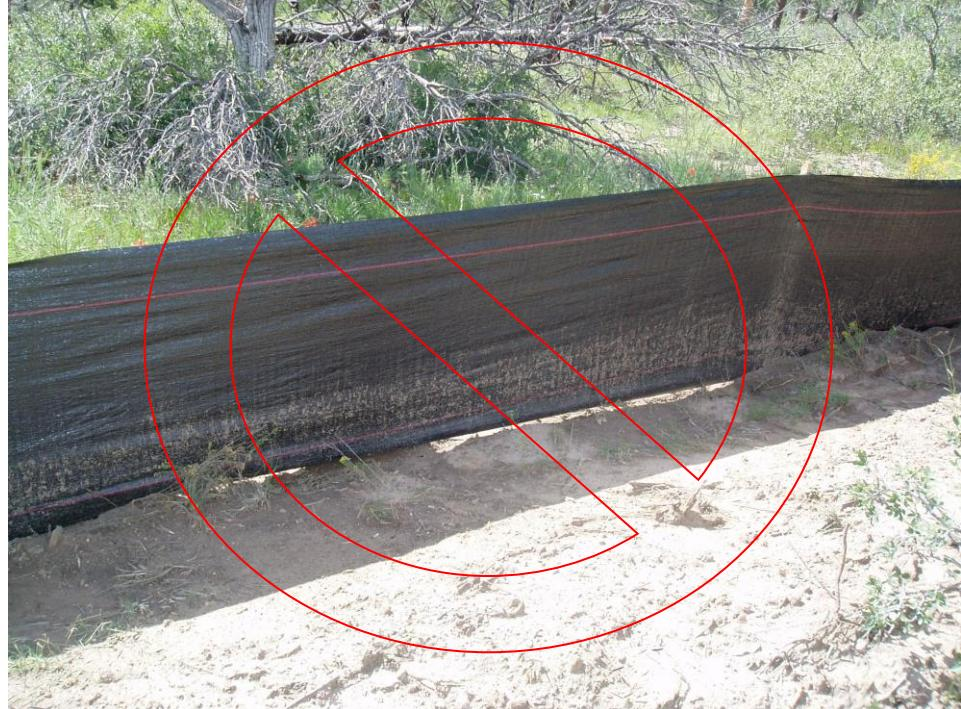
Silt fence should be properly entrenched for proper operation.
