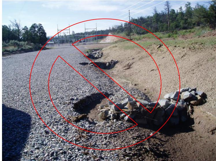
Notice how runoff bypassed the check structures. Channel banks must be sufficient to withstand flows and the dam center must be lower to allow flow over the check dam.
