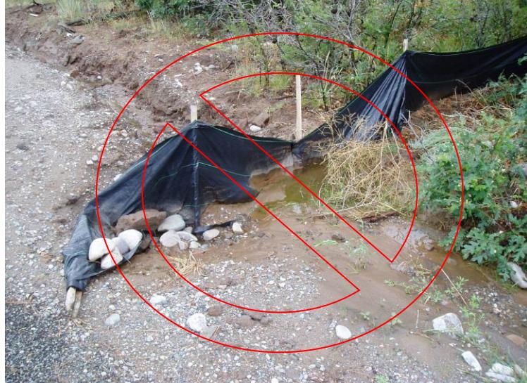
Silt fence cannot be used as a check structure and is not designed for concentrated flow.
