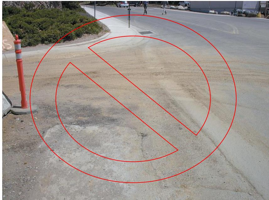
Failure to install a construction entrance has led to sediment transport offsite.
