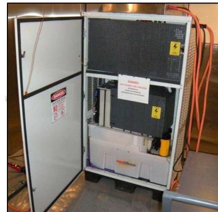
RedFlow 10kWh Zn-Br flow battery
