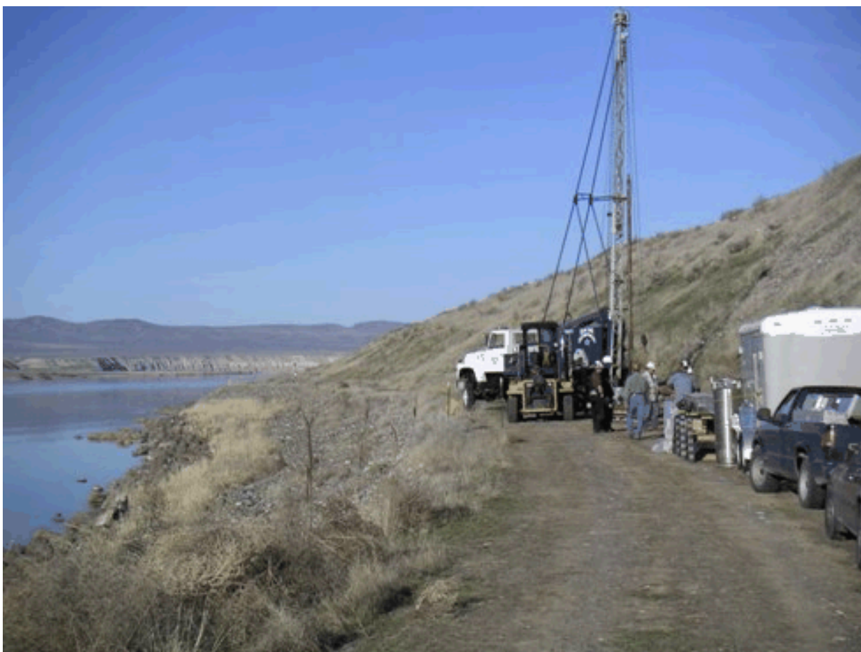
Figure 3 Drilling an injection well next to the Columbia River at the Hanford site.
