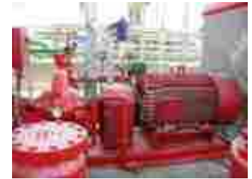
Motor Driven (Electric) Fire Pump
