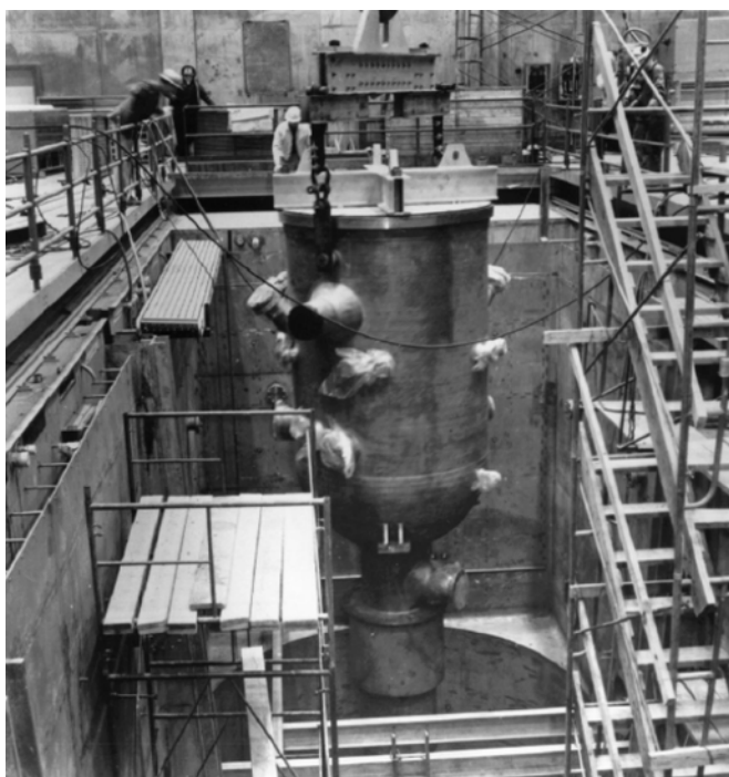
FIGURE A1.4. Original Installation of the HFIR Pressure Vessel. The HFIR building and pool were designed to support pressure vessel replacement.
