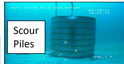
Figure 3. Scour pile deployed at anchor base II
