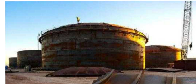
6 hours of molten-salt storage heated from ~300 - 400 C (1.7 GWh)
