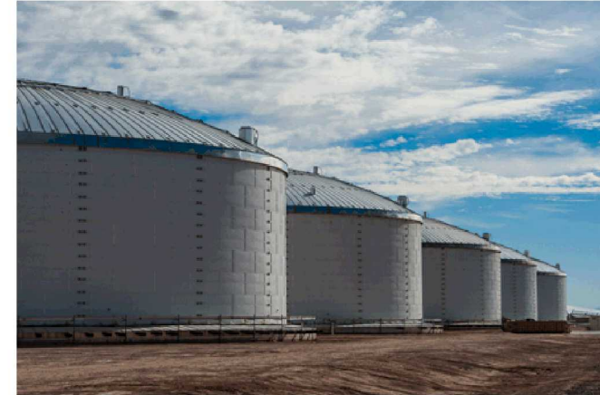
Molten-salt storage tanks at Solana CSP plant in Arizona. Credit: Abengoa
