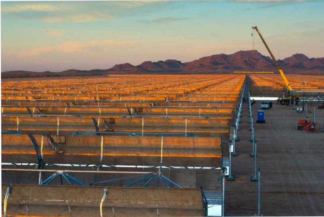
280 MW parabolic trough plant Phoenix, AZ (Gila Bend) Started 2013
