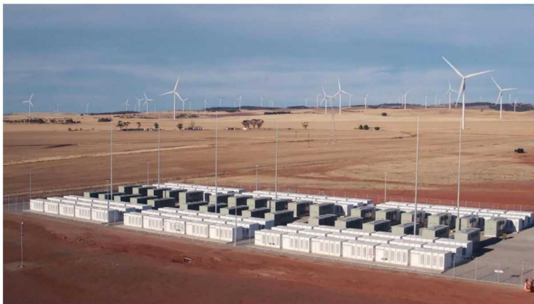
Tesla 100 MW / 129 MWh ESS Australia - Grid stability
