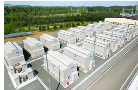
34MW /245 MWh NAS at a wind farm Rokkasho, Aomori, Japan (Source: NGK, 2017)
