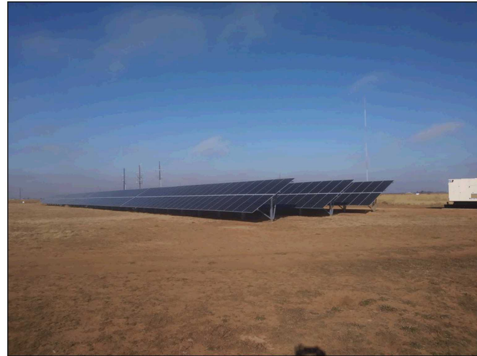
Figure 3: 150 kW Solar Array
