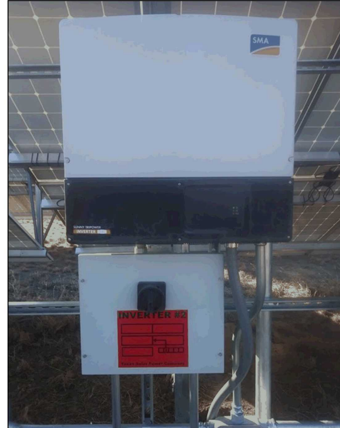
Figure 4: 30 kW Inverter
