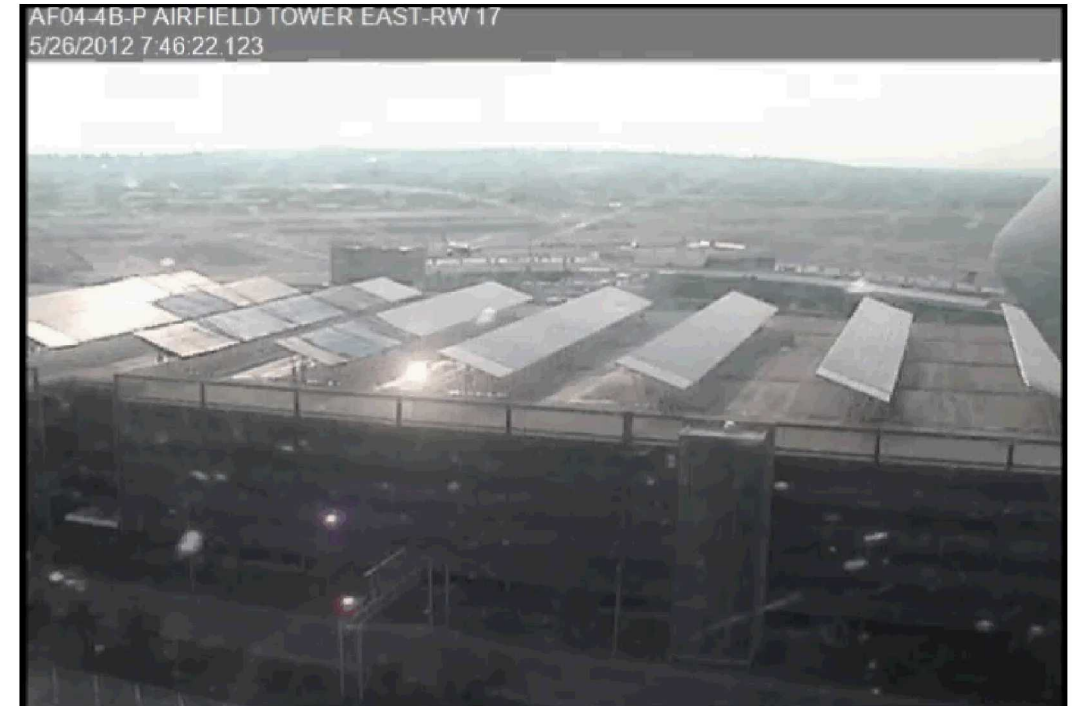
Glare observed from airport traffic control tower at Manchester-Boston Regional Airport (May 2012). The $3.5M array had to be tarped.
