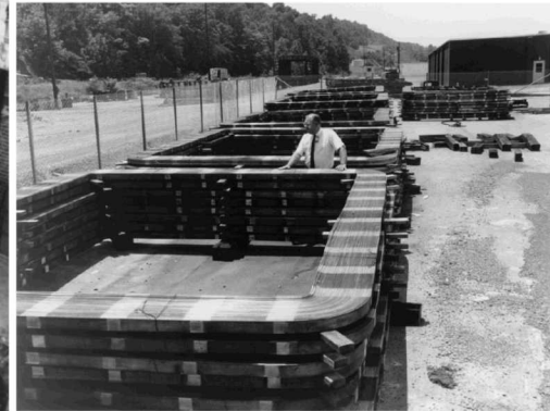
Figure 7. Calutron silver coils before return to U.S. Treasury. Photo source: Y-12 126949.
