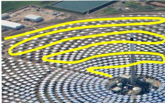
Assess field for optical errors using far-field targets
