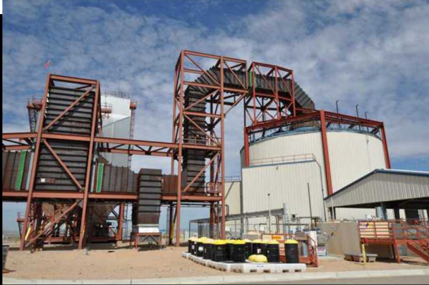
New Flame Facility
