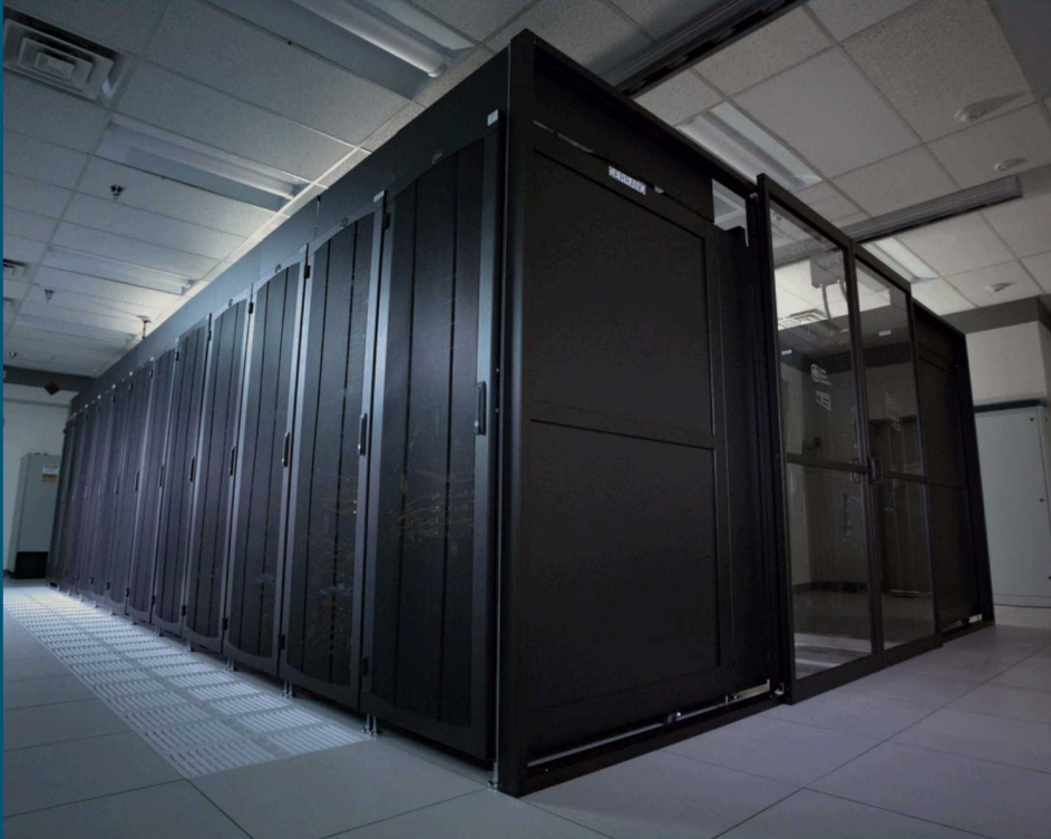
Typical Super Computer Cluster 80,784 compute cores 1.223 petaFLOP
