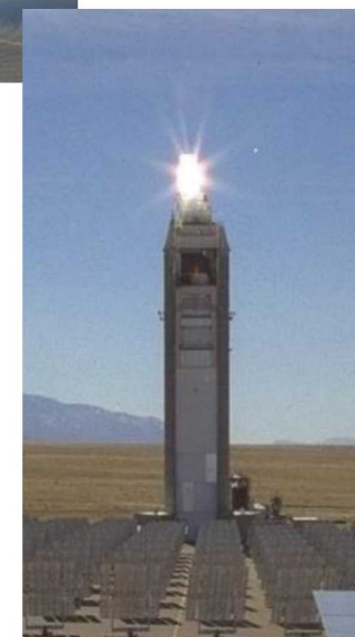
Thermal emission from receiver at ~600 C
