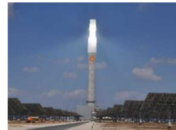
Gemasolar, molten salt, 19 MW e , Spain, 2011
