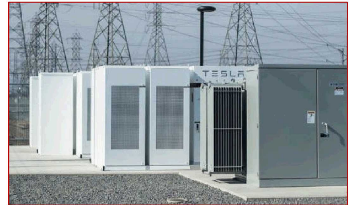
SCE/Tesla 20MW - 80MWh Mira Loma Battery Facility
