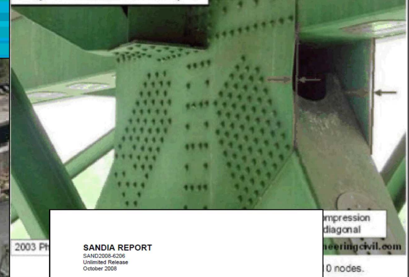
Gusset Plate Distortion (all four U10 Nodes)
