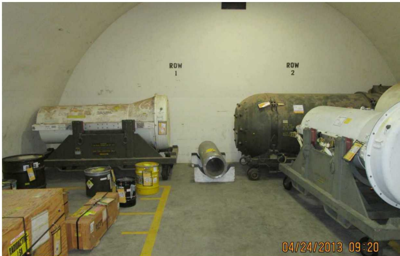
Monzano Alarm and Nuclear Material Consolidation Project
