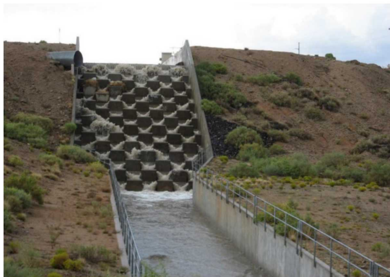
“Dragon’s teeth,” stormwater energy dissipater located south of SWSP-05.
