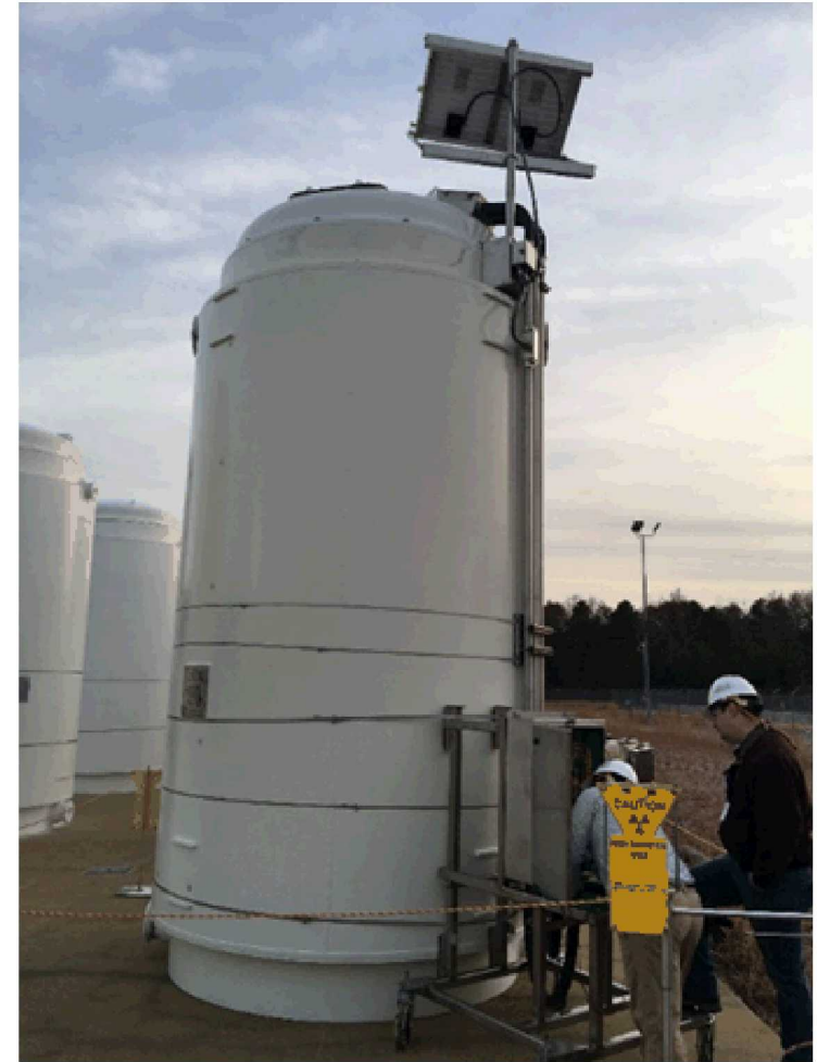
Photo courtesy of Dominion Energy
