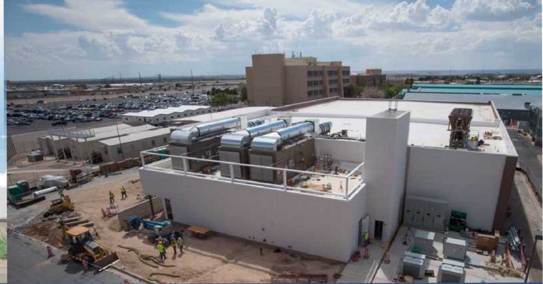
Construction Completed < 1 Year
