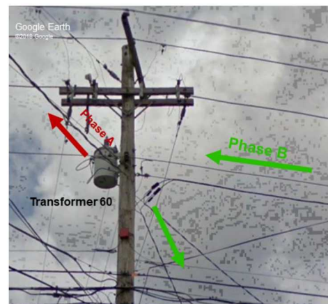
Figure 8 - Phase B from Transformer 61 serving another customer and Transformer 60 connected to Phase A
