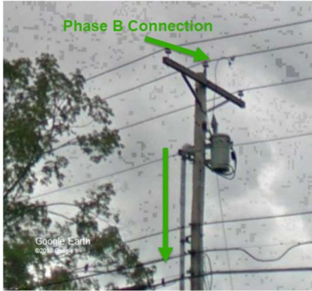
Figure 2 - Example of a phase labeling error with the correct phase being Phase B [14]
