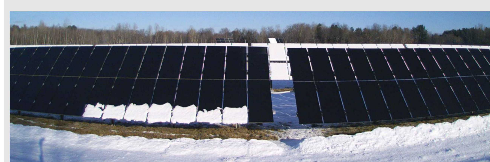
Snow shedding at different rates at 9:15 December 8, 2018. Note that 20% snow coverage causes significant energy losses.
