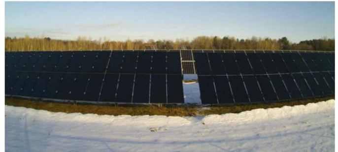
Fig. 1. Photograph of the two PV systems at the VT field site. Left modules are framed, right modules are frameless.
