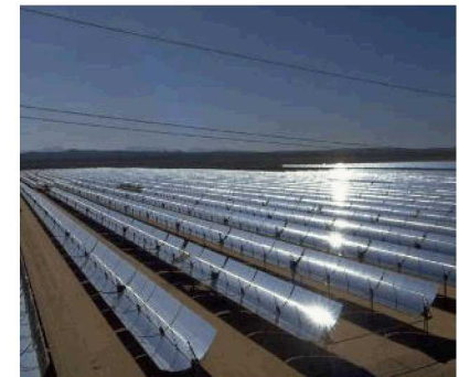
Parabolic Trough Collectors at Kramer Junction, CA
