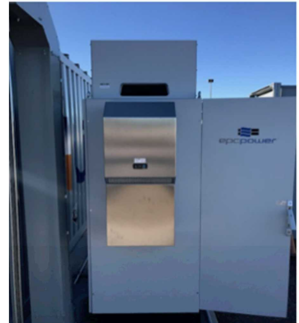
On board cooling system for EPC 125kW bi-directional inverter.
