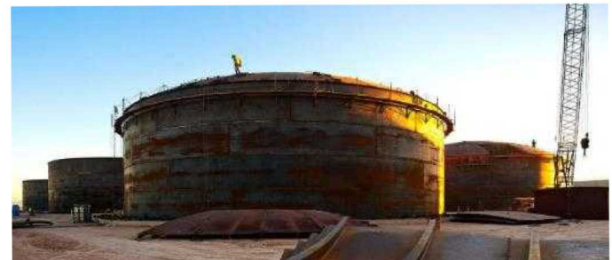
6 hours of molten-salt storage heated from \sim 300 - 400 C (1.7 GWh)
