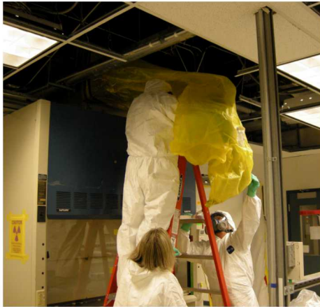
Removing old ducts and HEPA filters
