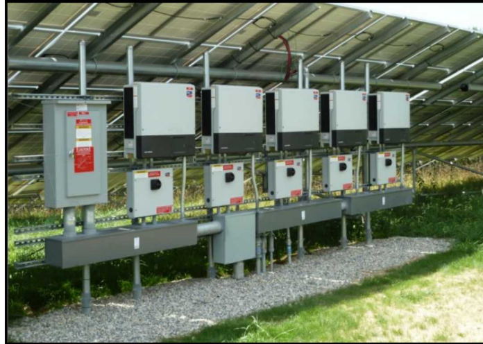
Figure 6-2. PV Inverters at the Old Upton Rd PV Site.
