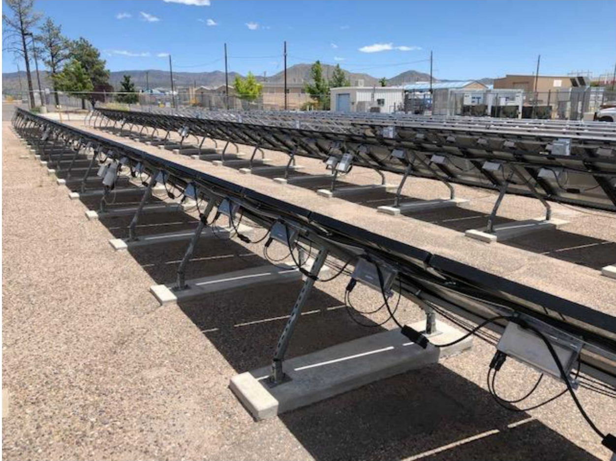
Figure 3-10: DETL East Array with 100 microinverters and 10 PVS5s.
