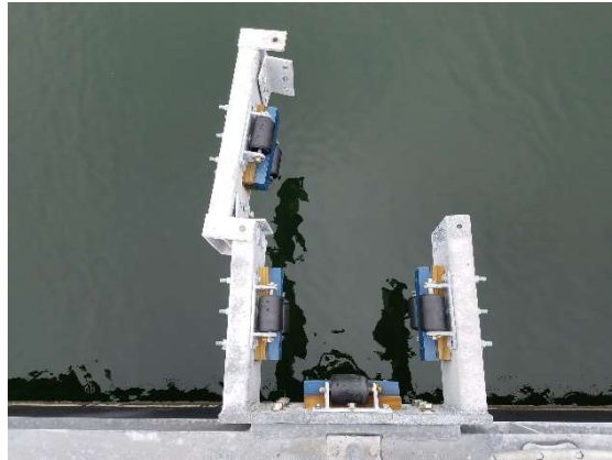
Figure 12. Mooring system for Tidal Energy Test Site at Memorial Bridge (Living Bridge Project). Custom-designed pile-guides with redundant rollers and additional redundancy recessed wear-blocks.
