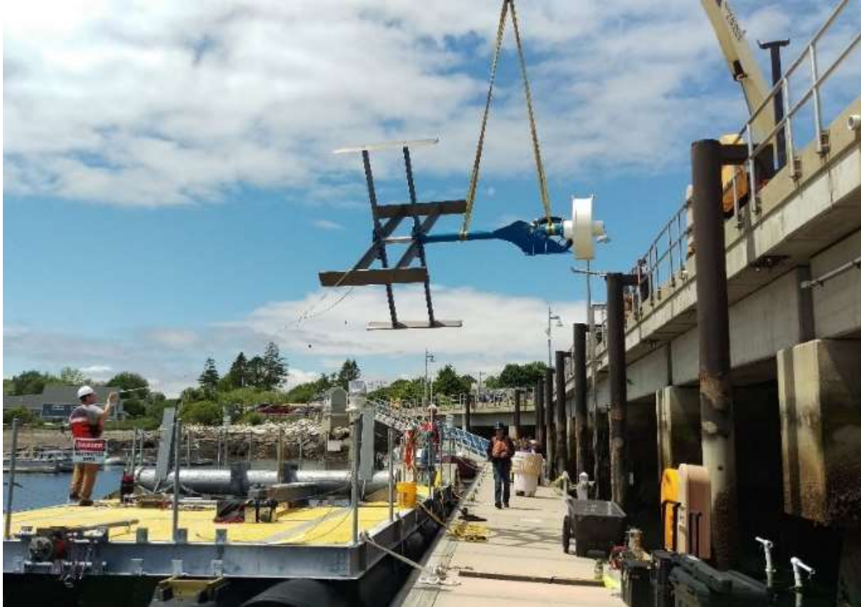
Figure 5. Tidal Turbine during installation on the TDP at UNH Pier.
