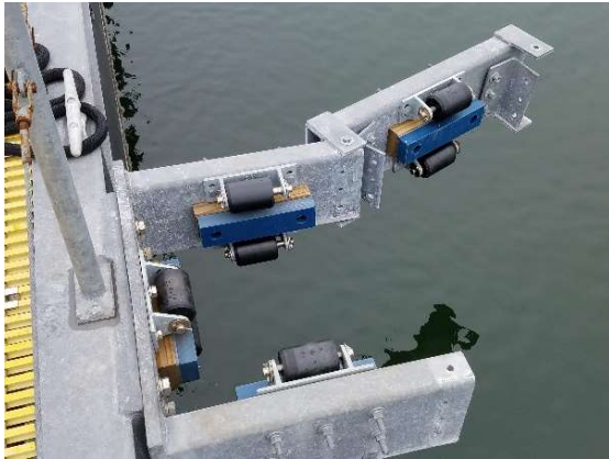
Figure 12. Mooring system for Tidal Energy Test Site at Memorial Bridge (Living Bridge Project). Custom-designed pile-guides with redundant rollers and additional redundancy recessed wear-blocks.
