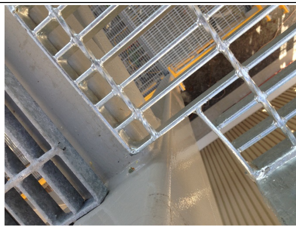
Exhibit 11.2. Example of Two Problems with the Cross-over Grating, 1) Lack of Support at Edges and 2) Gap Too Large Between Adjacent Pieces, 9/19/2014.
