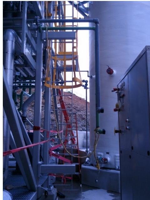
Exhibit 4.5.2. Secondary Egress Ladder Installation, 10/15/2014.
