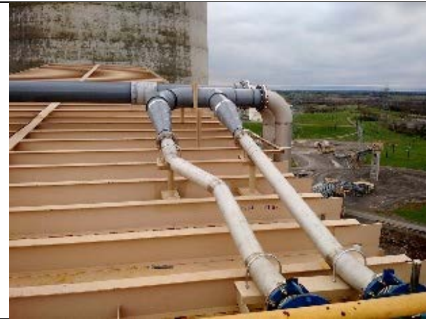
Exhibit 4.6.1. Flue Gas Supply Lines Installed at Top of Stack Duct, 4/7/2015.
