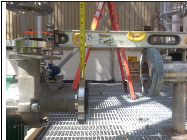
Exhibit 11.1. P-109 Connecting Pipe Section Did Not Fit Correctly, 9/30/2014.
