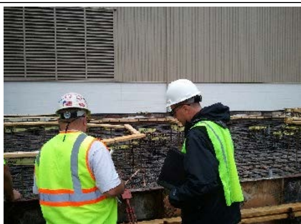
Exhibit 3.2.2. Reinforcing Steel Inspection by B+K During the Construction Phase.
