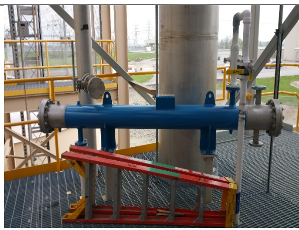
Exhibit 4.10.5. Heat exchanger (E-200) installation within Module 1.
