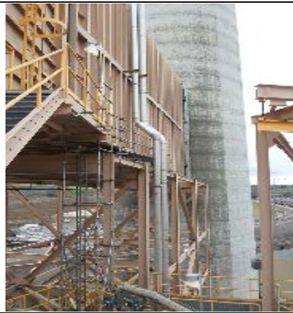
Exhibit 4.6.2. Vertical Sections of Flue Gas Supply and Return Lines, 4/7/2015.
