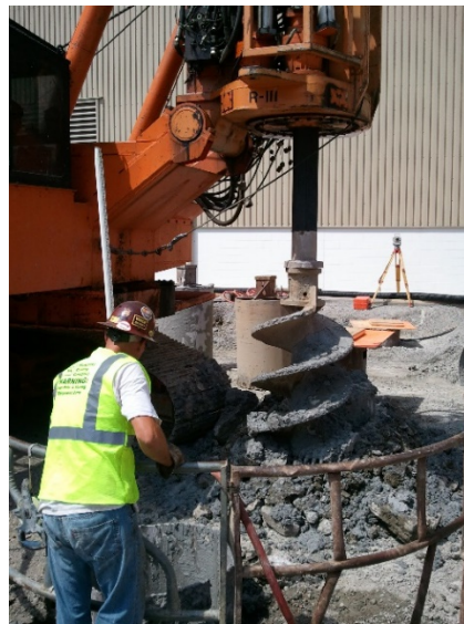
Exhibit 4.2.2. Drilling Foundation Pier A, 4, 6/13/2014.
