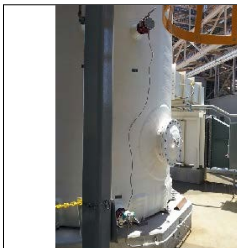
Exhibit 4.9.1. Cooling Tower Level Gauge (LT-C106-01), 5/7/2015.
