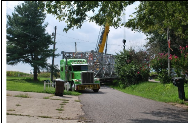
Exhibit 3.1.15. Shipping Modules Required a Crane to Lift the Back when Going Around this Corner, Very Near E.W. Brown Generating Station, 8/20/2014.
