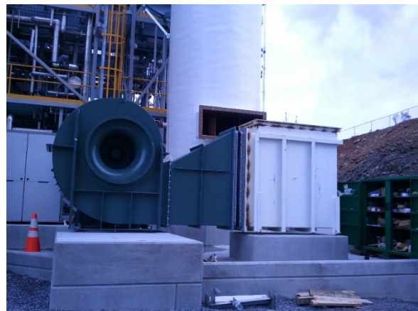
Exhibit 4.4.4. Cooling Tower Blower (B-103) is Set, 10/15/2014.
