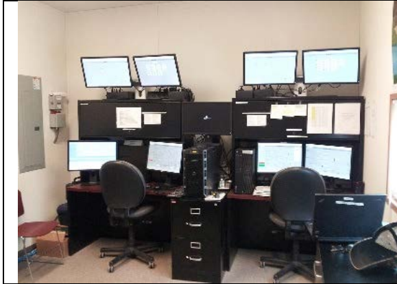
Exhibit 3.1.13. The Controlling Computers with Delta V Supplied by KMPS.
