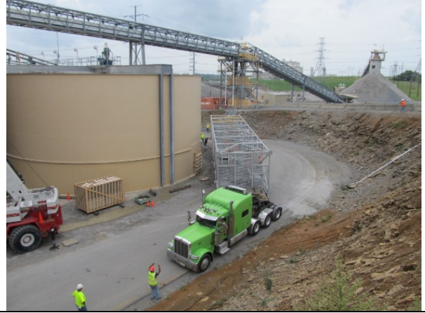
Exhibit 3.1.18. Moving Modules into Place for Erection at Process Site, 8/21/2014.
