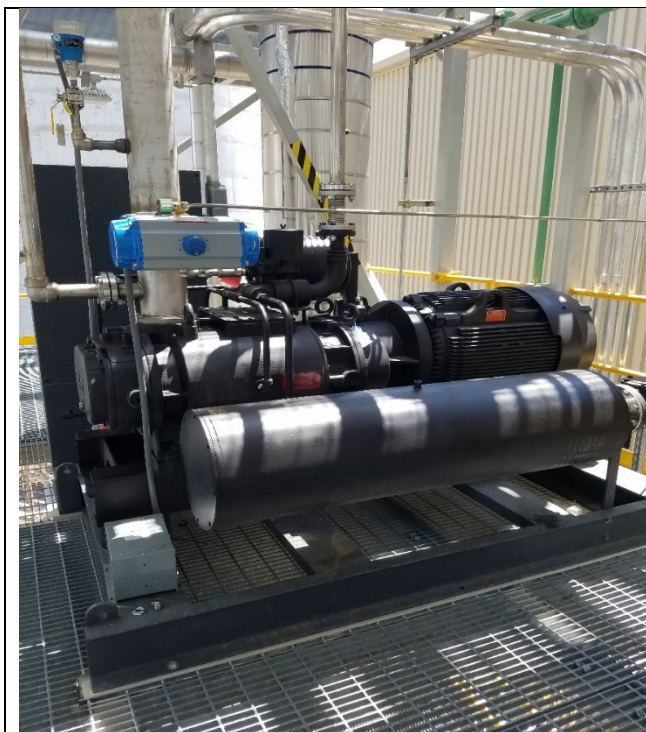
Exhibit 4.10.2. The vacuum pump installed within Module 2.
