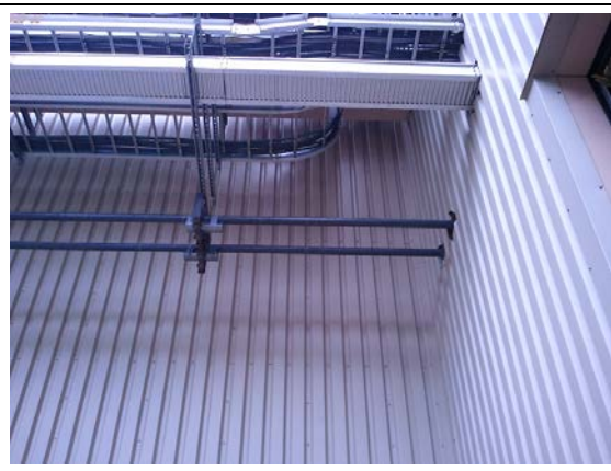
Exhibit 4.6.4. Steam Supply and Condensate Return Lines Installed on Pipe Roller Support, 12/3/2014.
