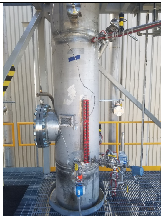
Exhibit 4.10.3. The solvent recovery column (C-200) installed within Module 1.
