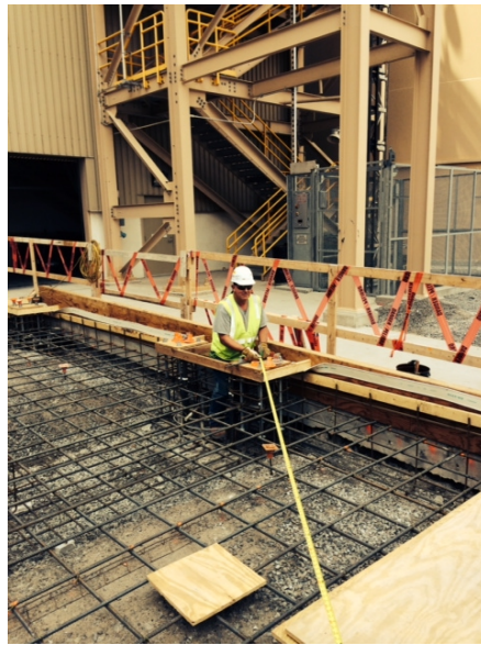
Exhibit 4.3.2. Modular Structure Anchor Bolt Dimension Check, 7/17/2014.
