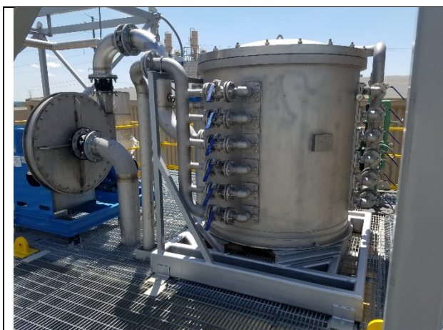
Exhibit 4.10.4. The MSU and B-200 blower installed on the newly constructed floor atop Module 2.
