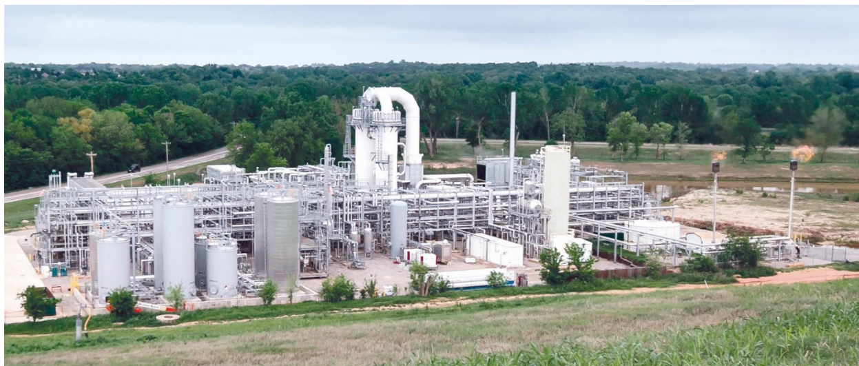
Figure 18. ENVIA's gas-to-liquids (GTL) plant in Oklahoma City, OK. From Voegelé (2017). Photo courtesy of Velocys.
