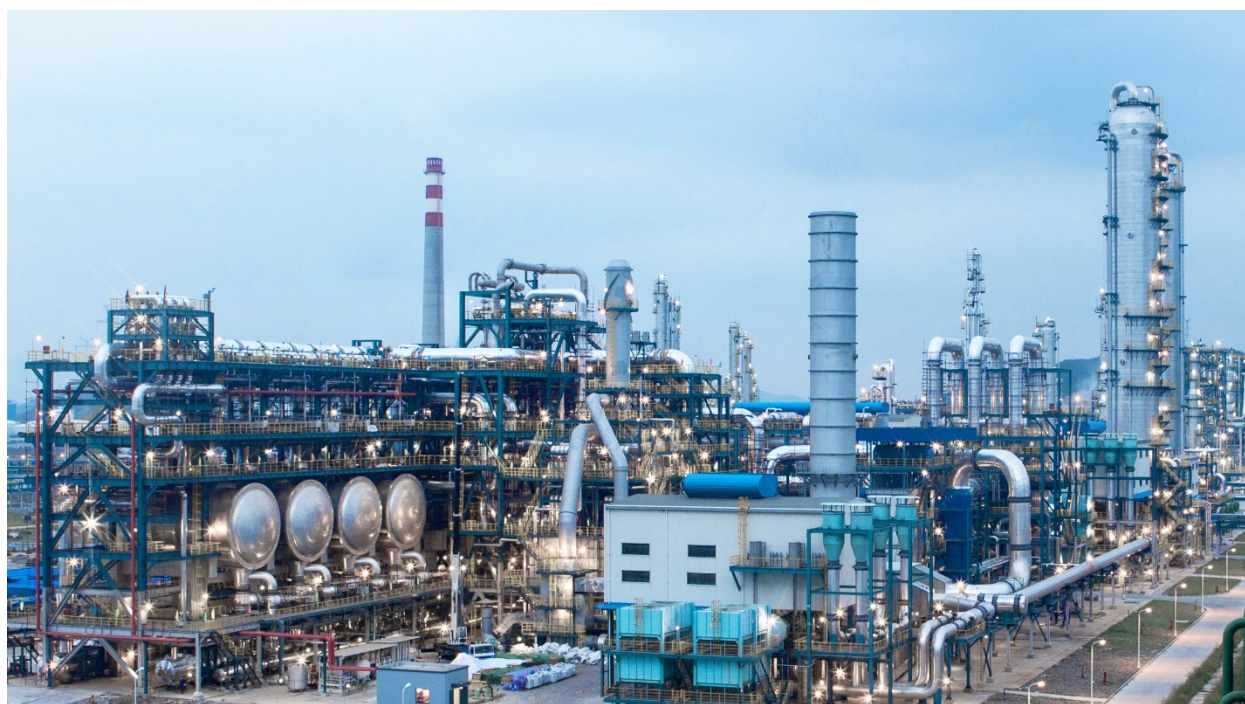
Figure 5. CATOFIN® propane dehydrogenation plant using Heat Generating Material at Ningbo Haiyue, China, Ningbo City, Zhejiang Province. (Photo courtesy of Clariant).
