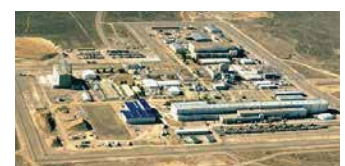
Naval Reactors Facility
