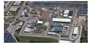
Savannah River Site
